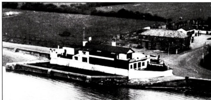
An aerial photo of the Boat House that shows the boat-shaped design.
